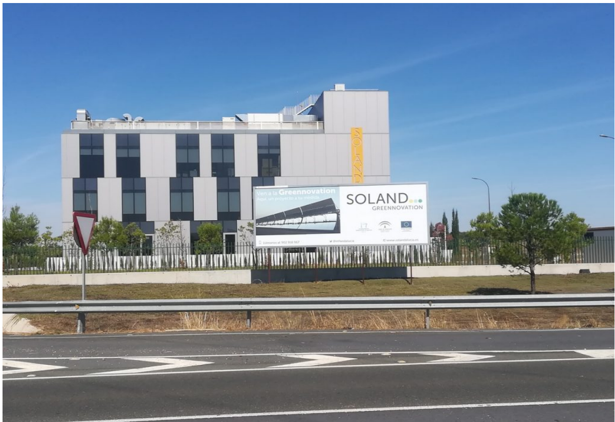
Le siège de Soland près de Sanlucar la Mayor. J'ai pas tout compris sur Soland, What is Soland. SOLAND is the new concept for a technology park of excellence developed by the Ministry for Economy, Innovation and Science of the Regional Government of Andalusia, with the help of the Innovation and Development Agency of Andalusia (IDEA), and the Council of Sanlúcar la Mayor. It is specifically focussed on renewable energies and eco-innovation.
